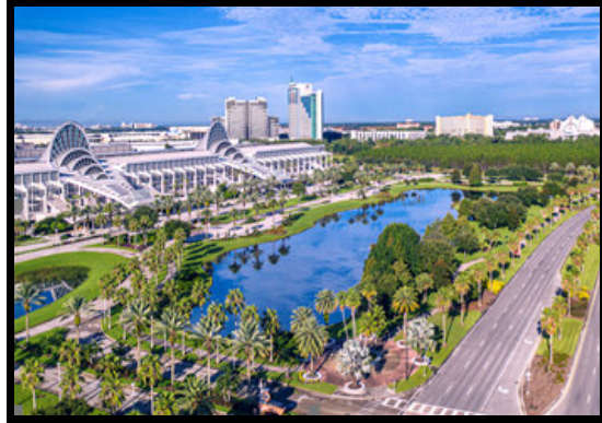
The OCCC North-South Building
